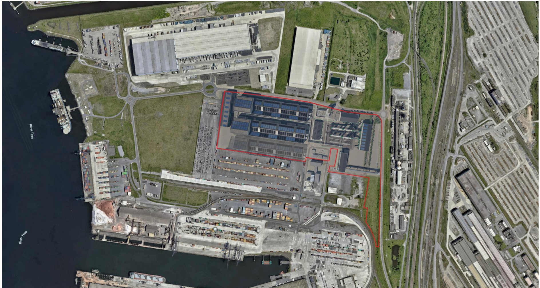
Figure 2.4 Rendered Aerial Image of site showing Proposed Development, with the third line transparent
