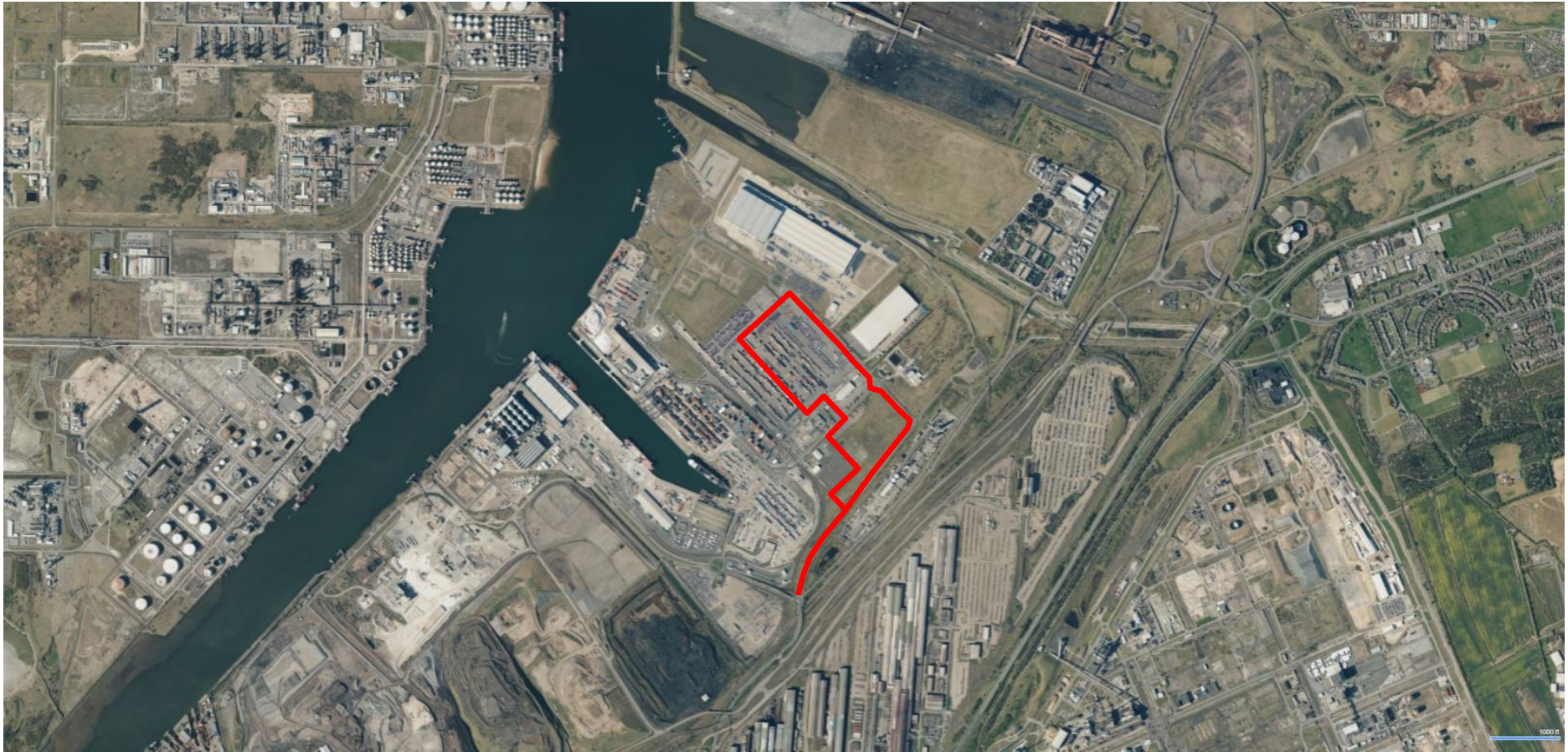
Figure 2.3 Site Location and Boundary (aerial view)
